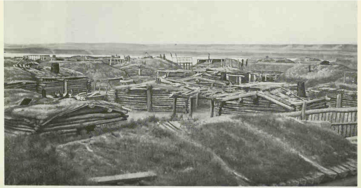
8. an hidatsa village in 1879—The original form of house was oval, dome-shaped, and covered with earth. A few of these can be seen in the background. The log cabins came in after white contact.
