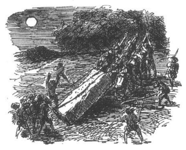
And this was the way they were heaving it along: The slab of rock was lying flat on the ground. Twelve men with pointed stakes pushed them under the edge of the rock and levered it about a foot off the ground. A much larger group of men pushed much
