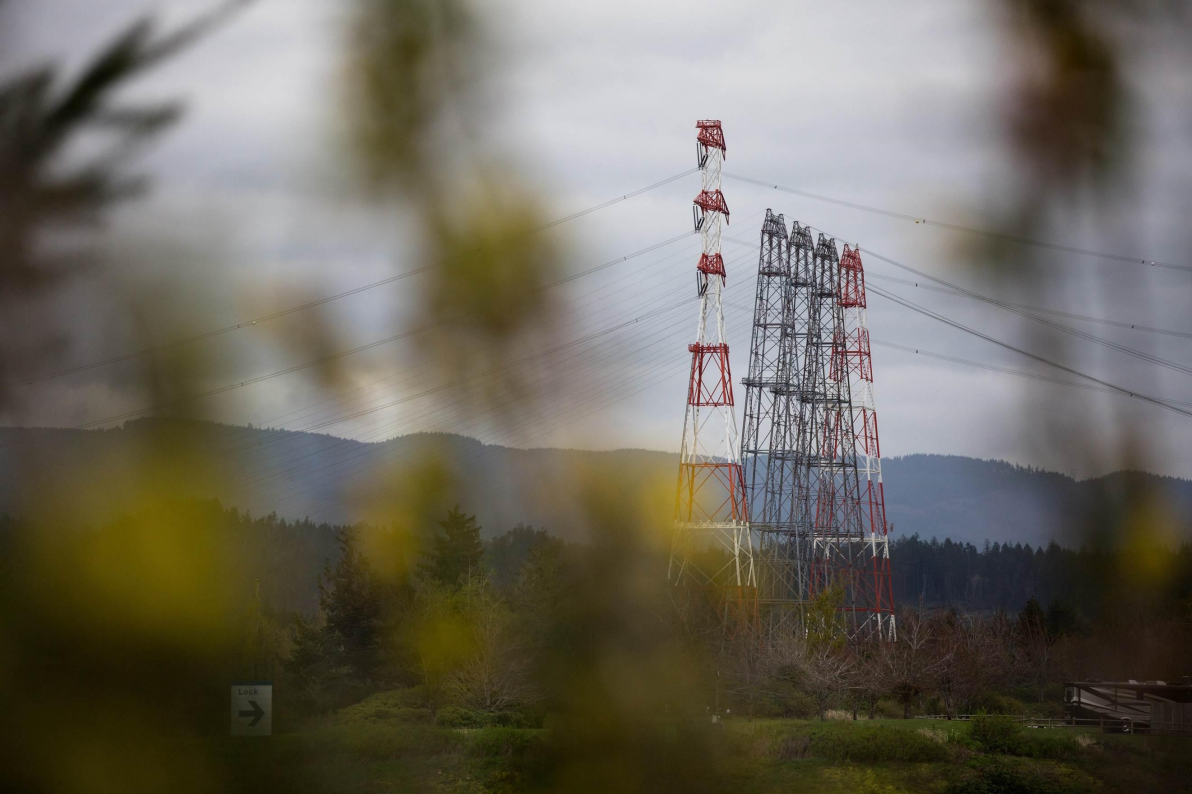
Four electrical substations in the Pacific Northwest were attacked in recent weeks. Substations convert high-voltage electricity that travels across long-distance transmission lines to the lower voltages used by businesses and residences. Pictured: Bonneville Dam power lines. Bradley W. Parks / OPB
