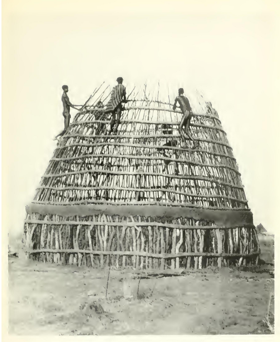
Building a cattle byre (Eastern Jikany)
