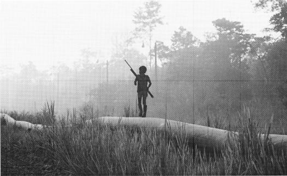
Along the pipeline
