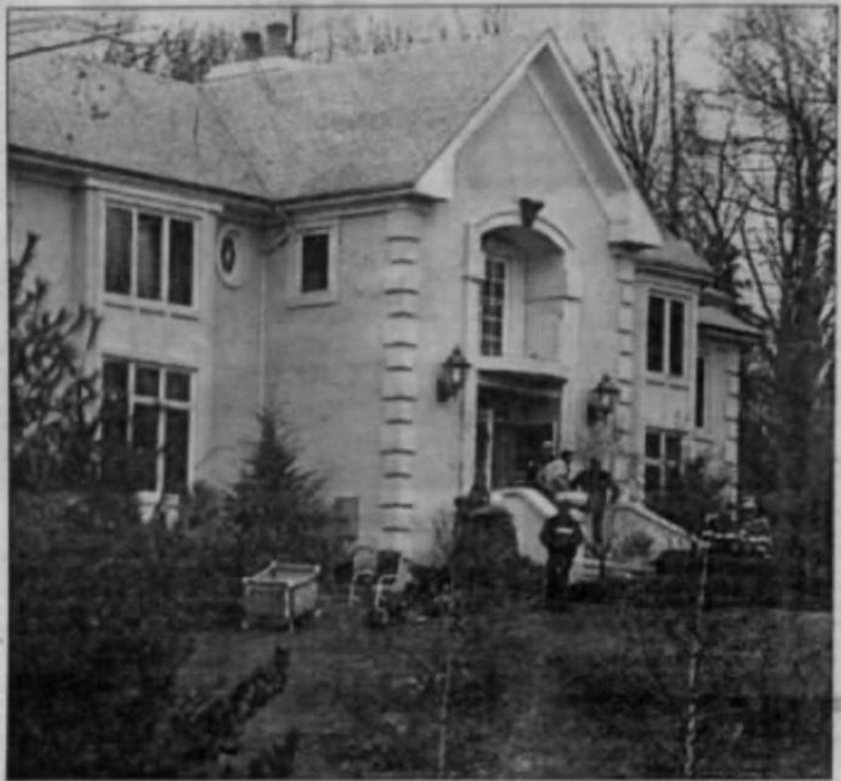
Emergency Workers and Essex County bomb squad crew examine home of THomas Mosser, who was killed by mail bomb in the North Caldwell, N.J., home yesterday.
